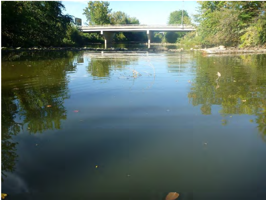
Photograph 5. Centennial Park Dam, Dam 1B Site, Blanchard River downstream.
