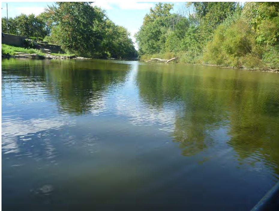
Photograph 20. Karg Dam, Dam 3B Site, Blanchard River downstream.
