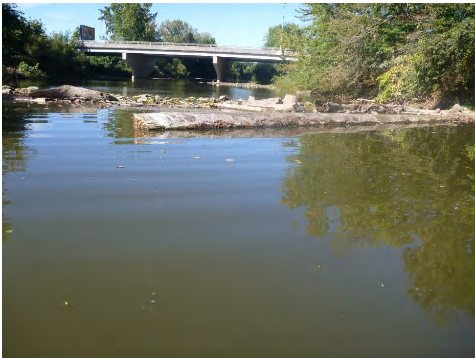
Photograph 8. Centennial Park Dam, Dam 1C Site, Blanchard River downstream.
