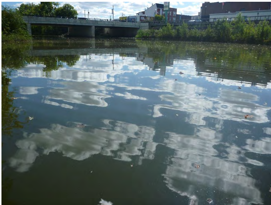
Photograph 10. Cory Street Dam, Dam 2A Site, Blanchard River upstream.
