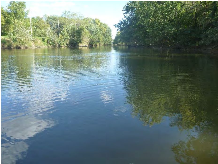
Photograph 25. Swale Park Dam, Dam 4A Site, Blanchard River upstream.
