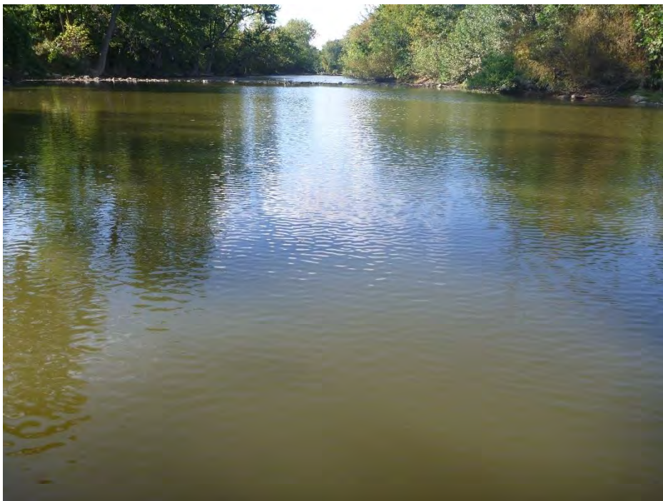
Photograph 26. Swale Park Dam, Dam 4A Site, Blanchard River downstream.
