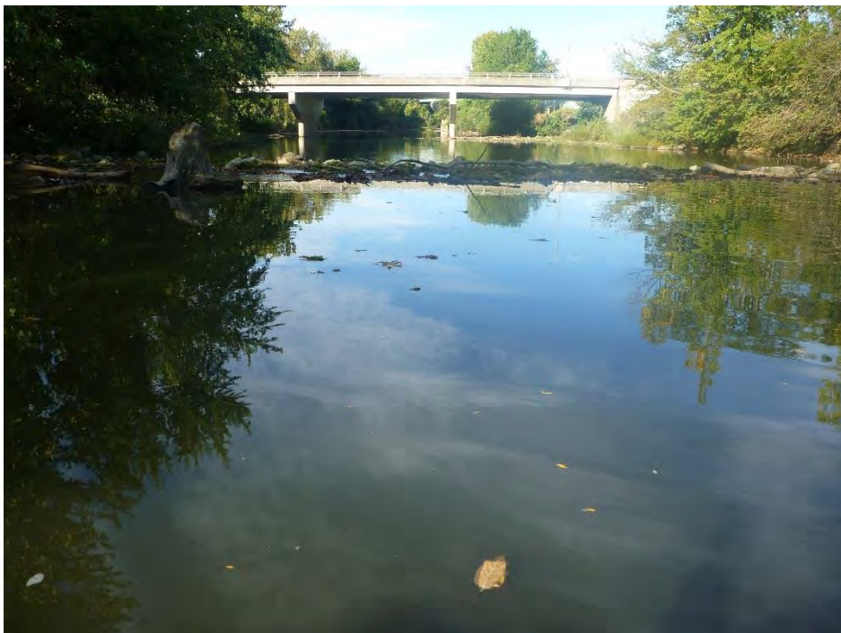
Photograph 2. Centennial Park Dam, Dam 1A Site, Blanchard River downstream.
