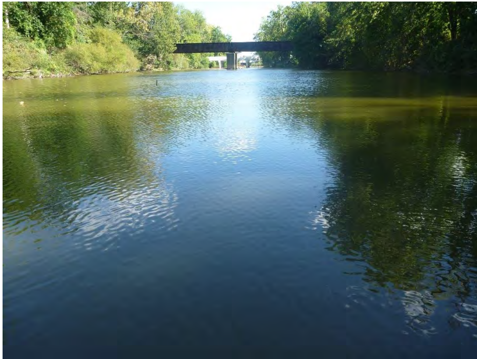
Photograph 19. Karg Dam, Dam 3B Site, Blanchard River upstream.
