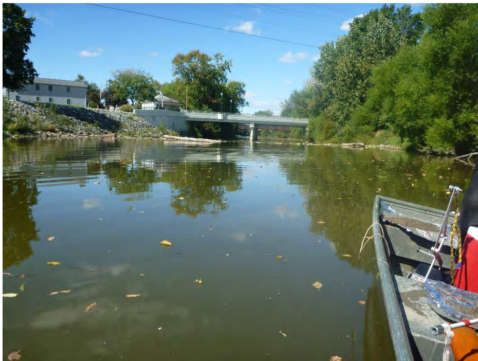
Photograph 14. Cory Street Dam, Dam 2B Site, Blanchard River downstream.
