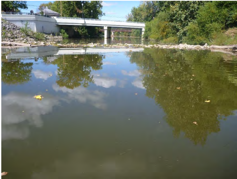
Photograph 11. Cory Street Dam, Dam 2A Site, Blanchard River downstream.
